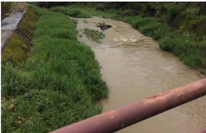
Photograph 3: View from the Shinkai Bridge to the down stream on 3 July 2022
